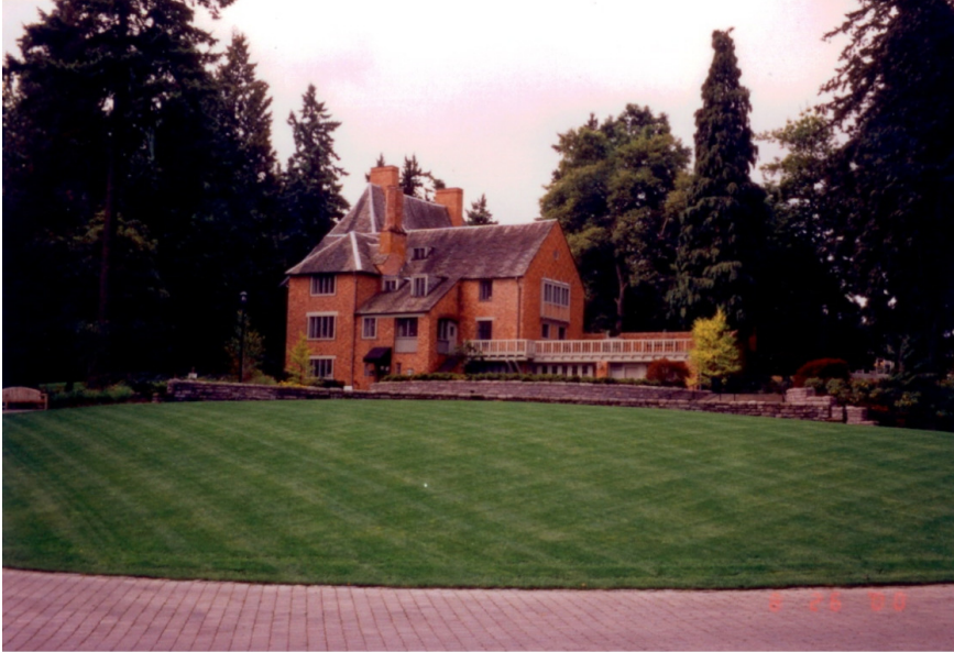
Vehicular Unit Paver Roadway, Grading, Lawn & Planting
