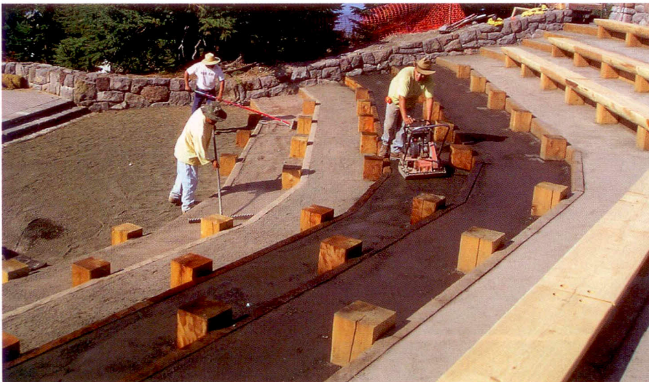
Thirty-foot-long cedar logs were placed on a lathe to be cut into precisely dimensioned rounds, top left. A bench mock-up displays the “draw knife” finish, top right, and the placement of the benches is shown in section, above. Cascadian Landscapers applied a gravel/pumice surface before attaching the benches, below.
